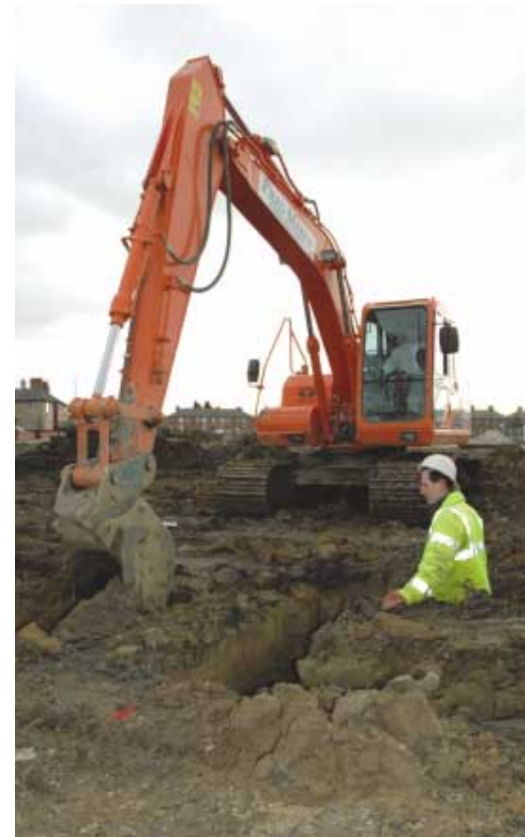
Foundation work well underway at Cleadon Park.
