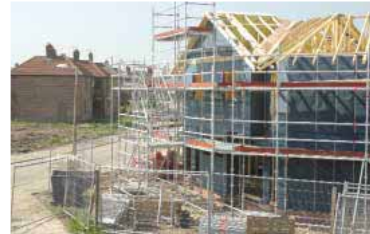
With the timber frame construction well underway, and sub contractors
